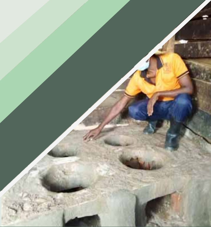
Energy saving cook stove being built by one of the CS in Rukungiri Bugangari cluster
